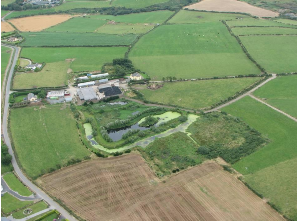
Figure V.1. Example of a constructed wetland downstream from a farmyard in Ireland. Photo: Harrington.
