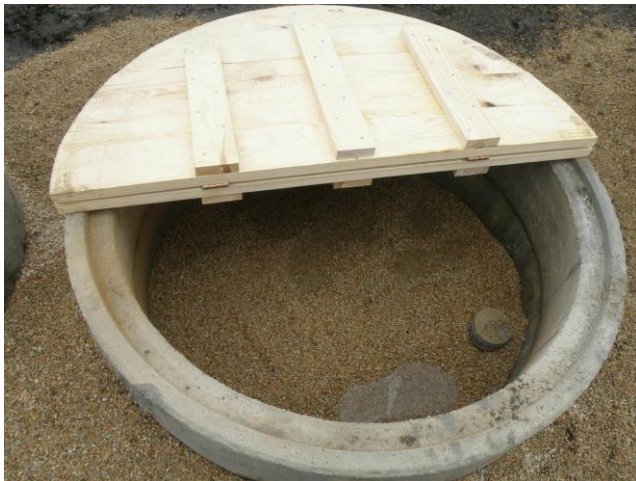
Figure V.9. Well with filter material receiving agricultural water. Photo: Piotr Nawalang.
